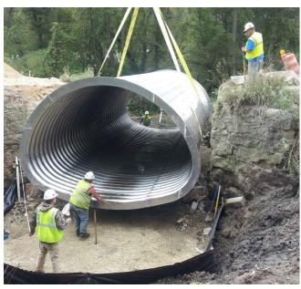
The Town of Onalaska in La Crosse County was seeking the replacement of four area bridges, however while working with GEC engineers, the Town opted to replace the bridges with culverts, at a fraction of the cost.
