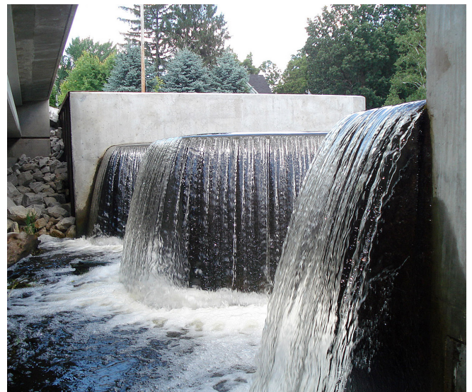
Town of Oconomowoc, Waukesha County, Monterey Dam
